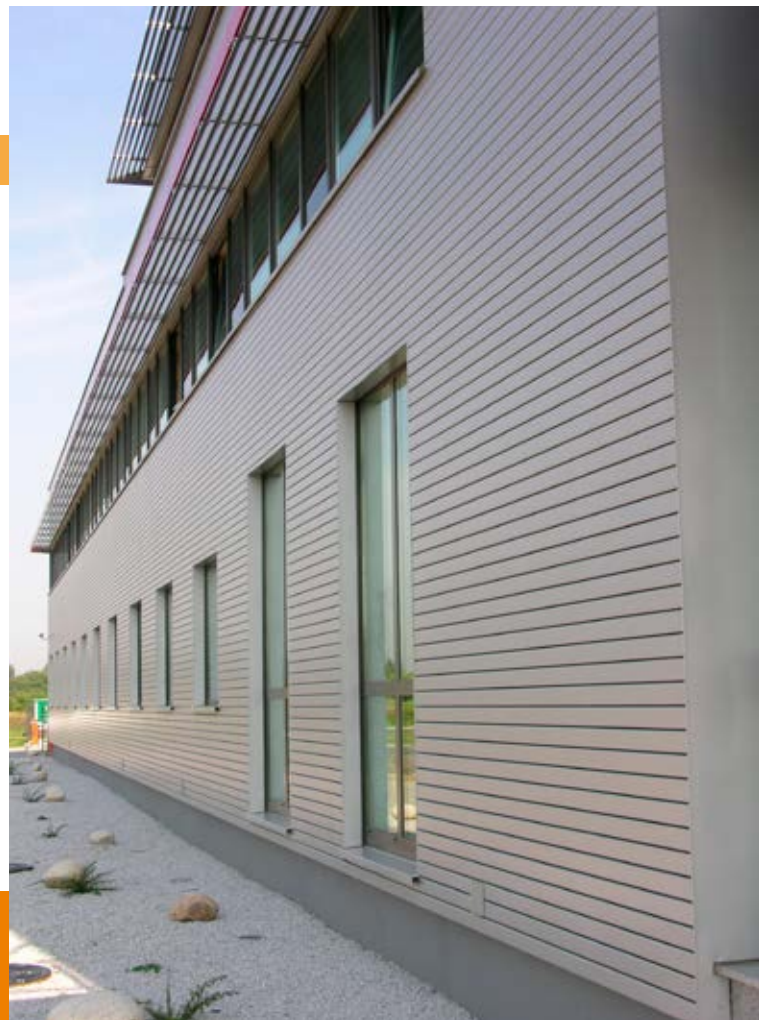
Panele S/84 na trawersynie T/u (szczelina pomiędzy panelami 16 mm) S/84 panels on T/u carrier (gap between pannels 16 mm)
