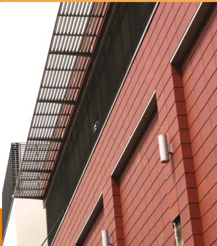
Panele S/84 na trawerszynie T/20 S/84 panels on T/20 carrier
