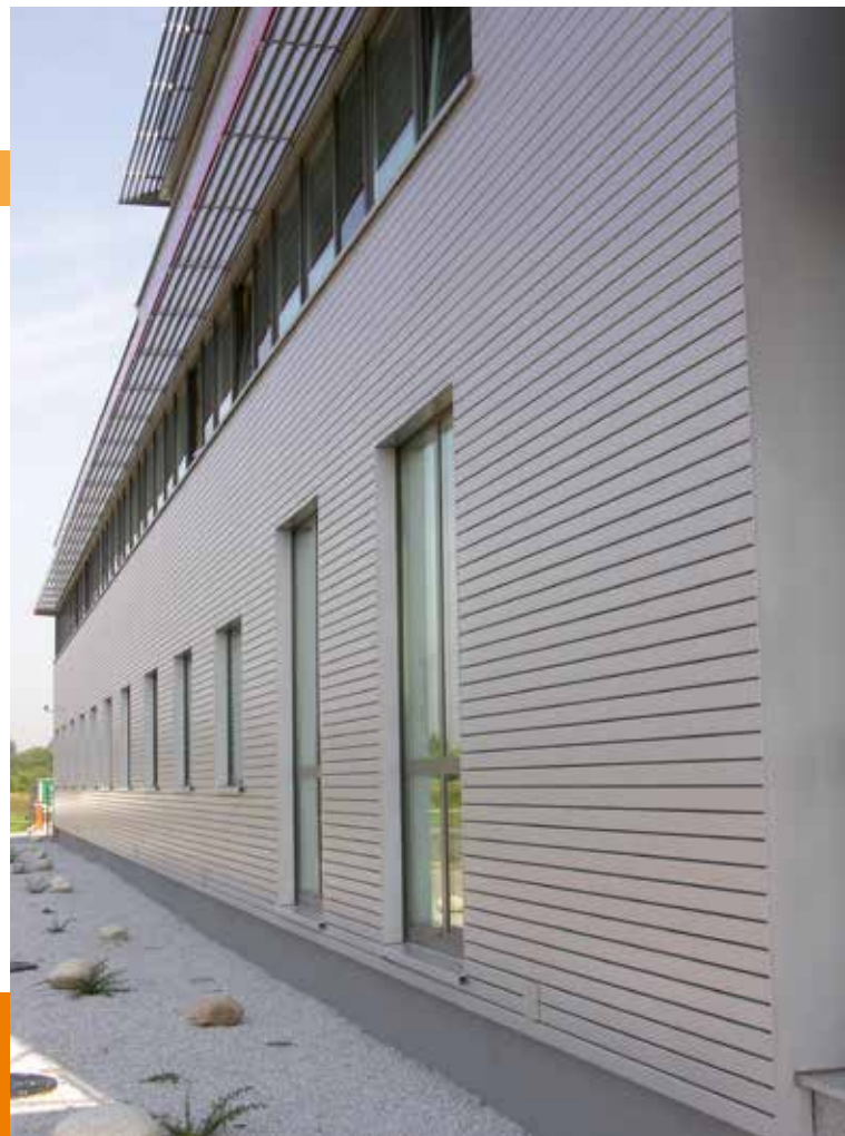
Panele S/84 na trawersynie T/u (szczelina pomiędzy panelami 16 mm) S/84 panels on T/u carrier (gap between panels 16 mm)
