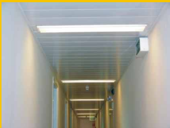
Sufit z paneli Omega 200
